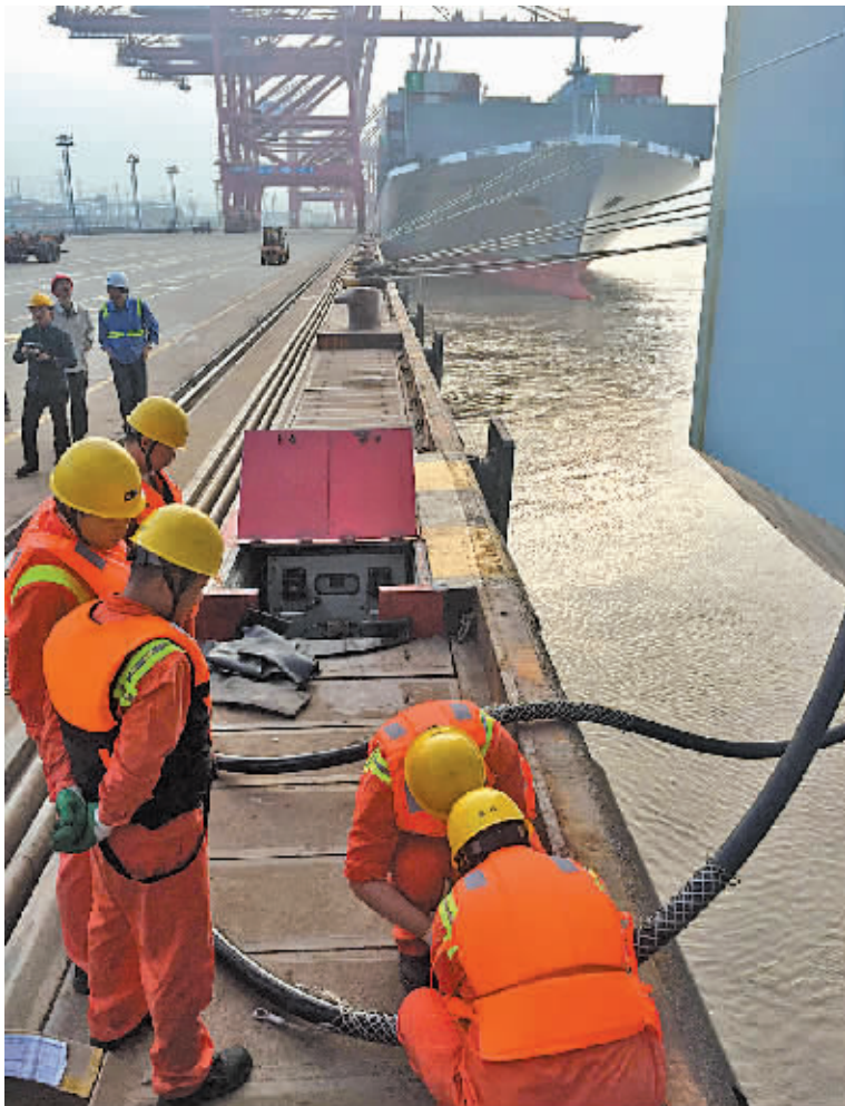
“中远丹麦”轮靠泊接岸电现场。(冯璋 王幕宾 摄)
