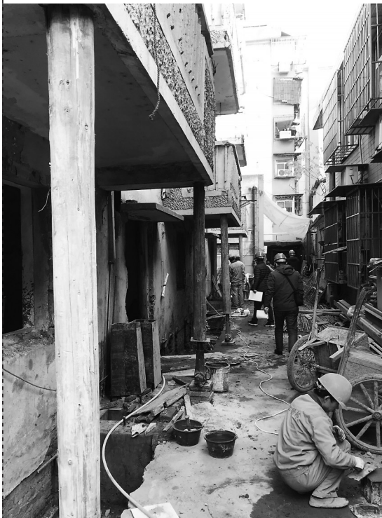
施工时,阳台用木柱支撑。
